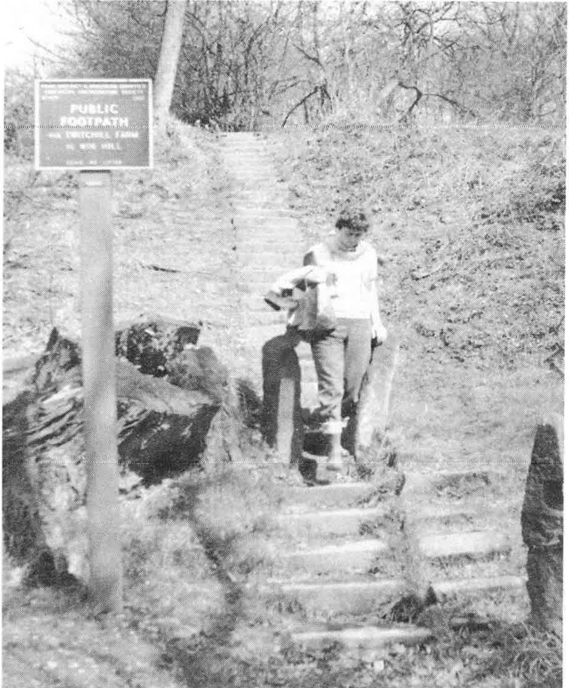
Old Footpath over Railway on Fullwood Lane
